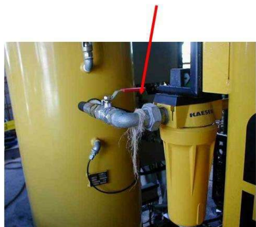
Pipe rope instead of pipe dope.
